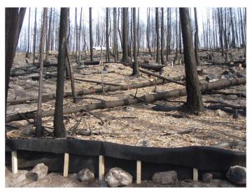
Photo 1. Sediment fence installation
