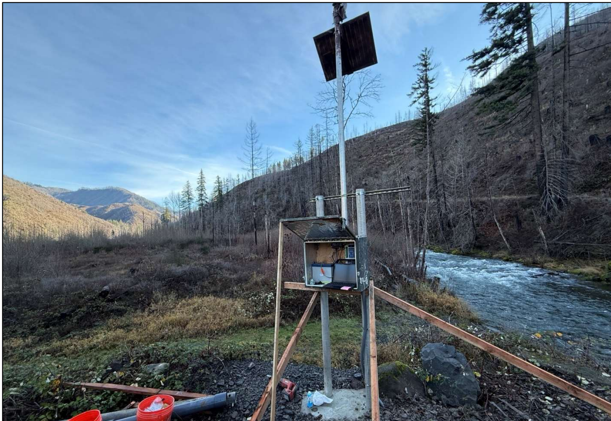
Figure 11-1: Installing New Upper Quartz Creek Water Quality Monitoring Station (USGS/EWEB)
