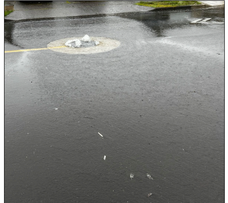
Sewer overflow at Daisy and S. 49 th Place on March 16 th , East Springfield
