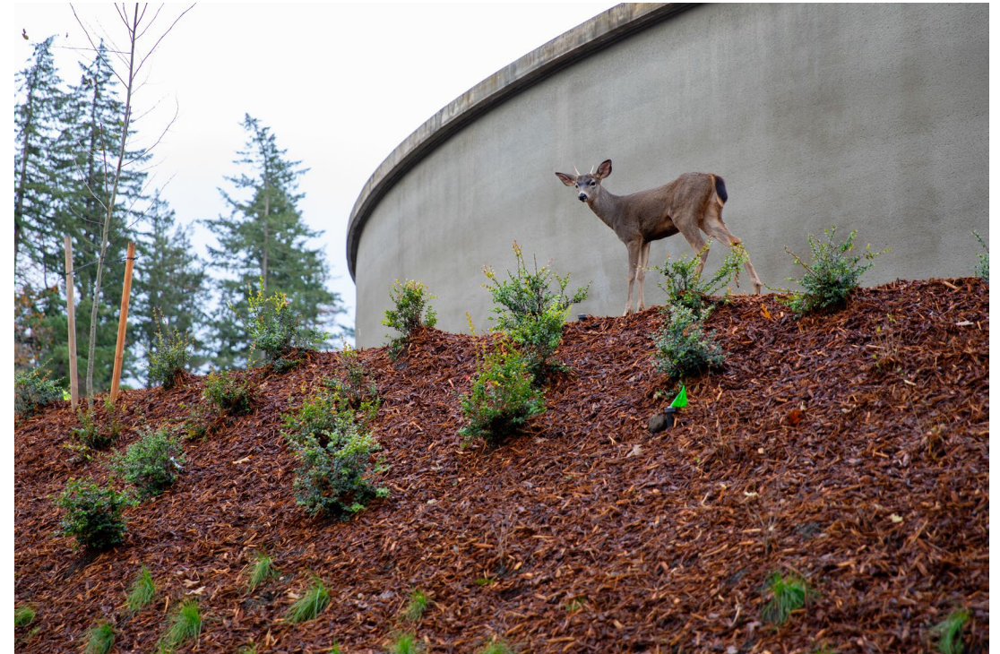
Similar cost control methods were used throughout the construction of the new E. 40 th water storage tanks.
