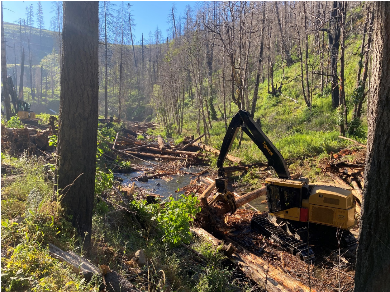
Figure 1-2: Gate Creek Large Wood Placement
