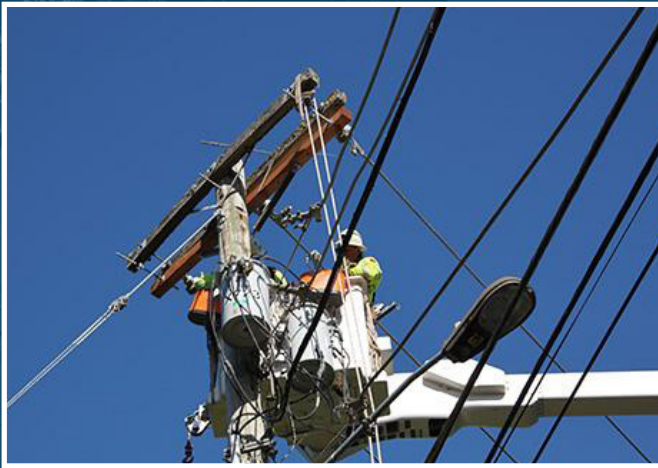
Crew member replacing cross-arm in 2021.
