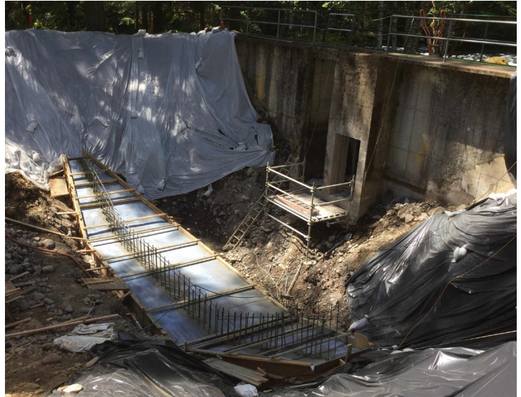
Construction of new salmon spawning channel exit.
