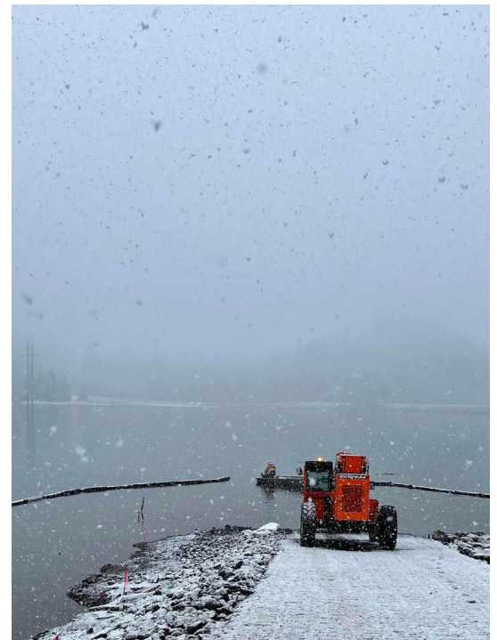
Construction of new boat ramp at Trail Bridge Campground was completed in December 2021 amidst snow flurries.
