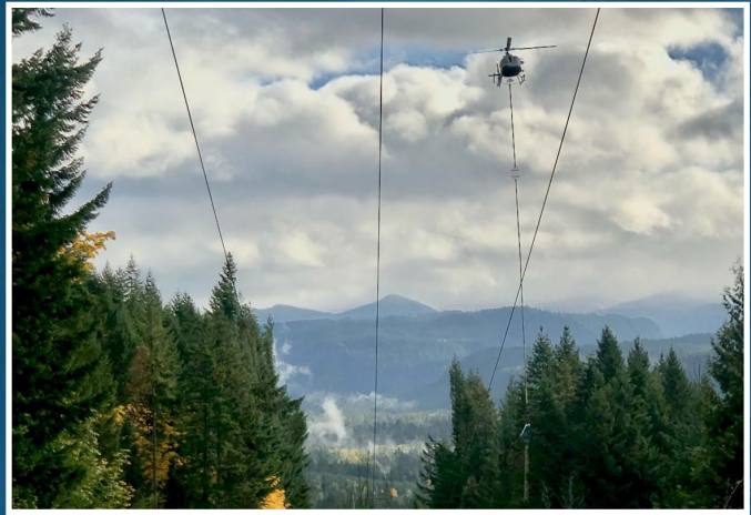
Aerial trimming of 12.5 miles along the Carmen-Smith transmission line.
