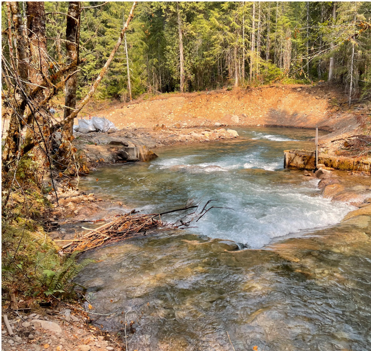
Improvements were made to the entrance of the salmon spawning channel below Trail Bridge Dam.
