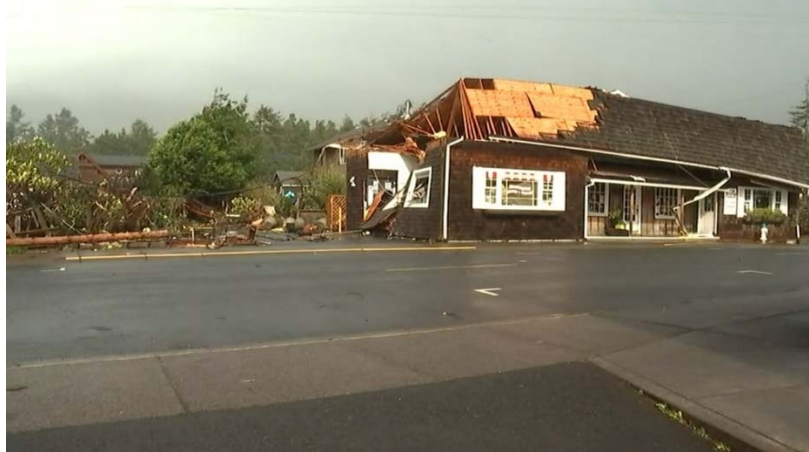
Picture 2-1. Source: KPTV-Manzanita, Oregon tornado damage October 2016
