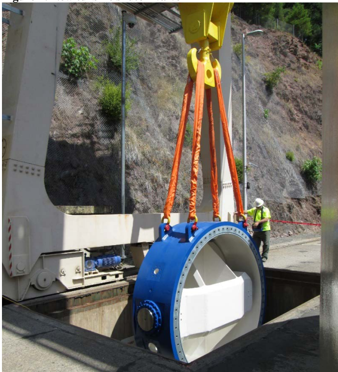
Figure 4: New turbine shutoff valve
