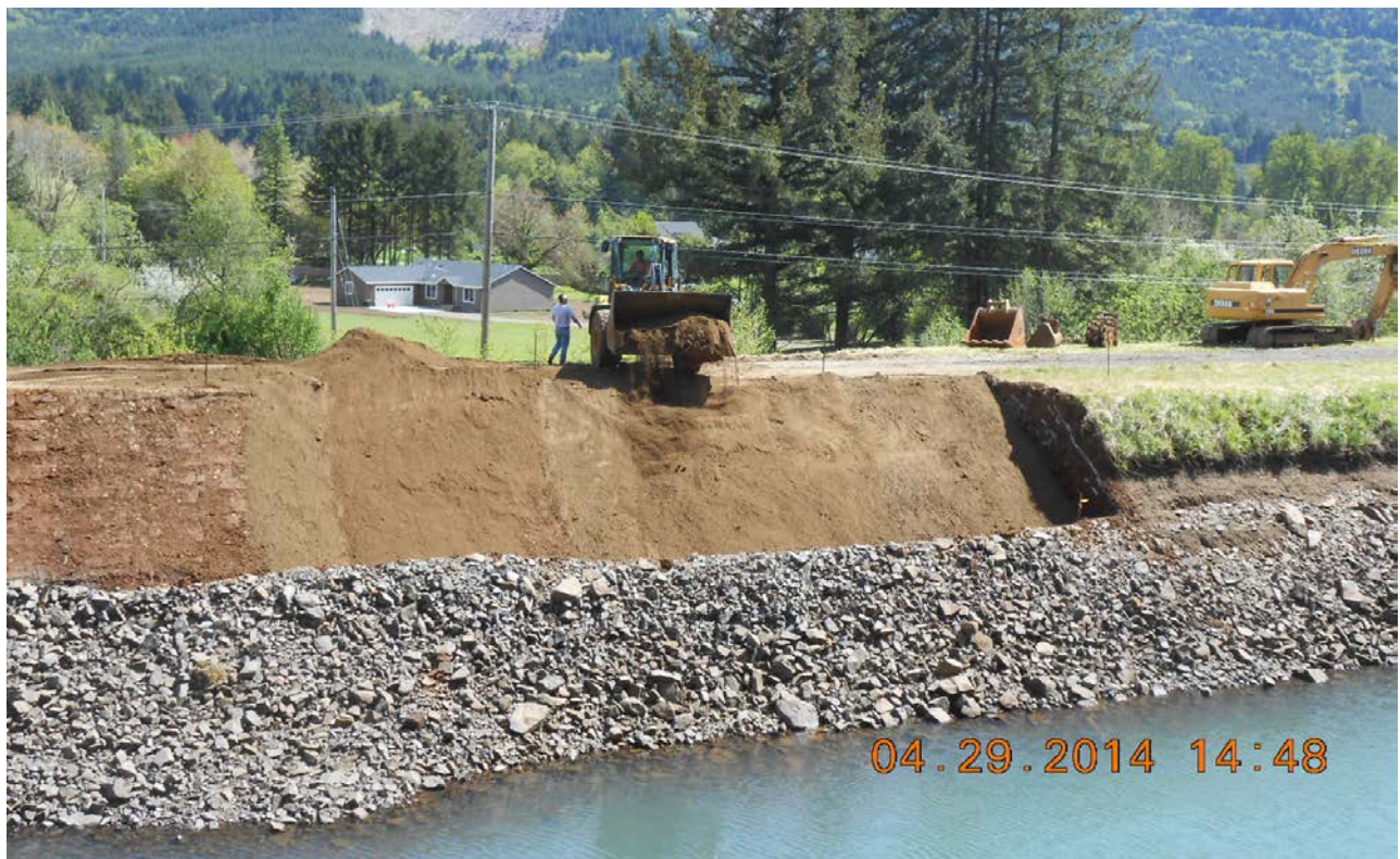
Figure 4. Shallow canal slope repairs, Leaburg Canal 2014
