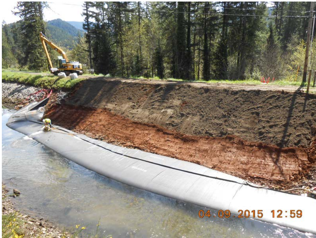
Figure 5. Deep canal slope repairs with coffer dam, Leaburg Canal 2015
