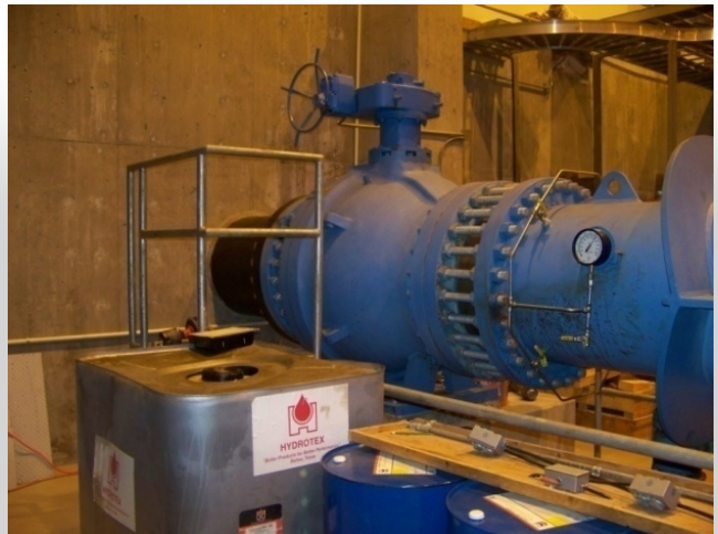
Typical Unit Penstock Penetration into Powerhouse
