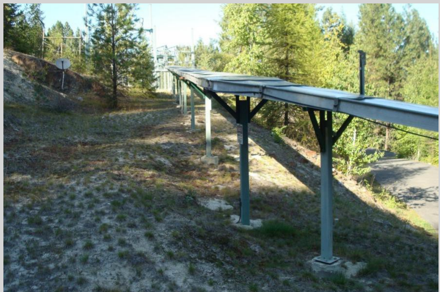
Generator Lead Raceway (Wire Tray)
