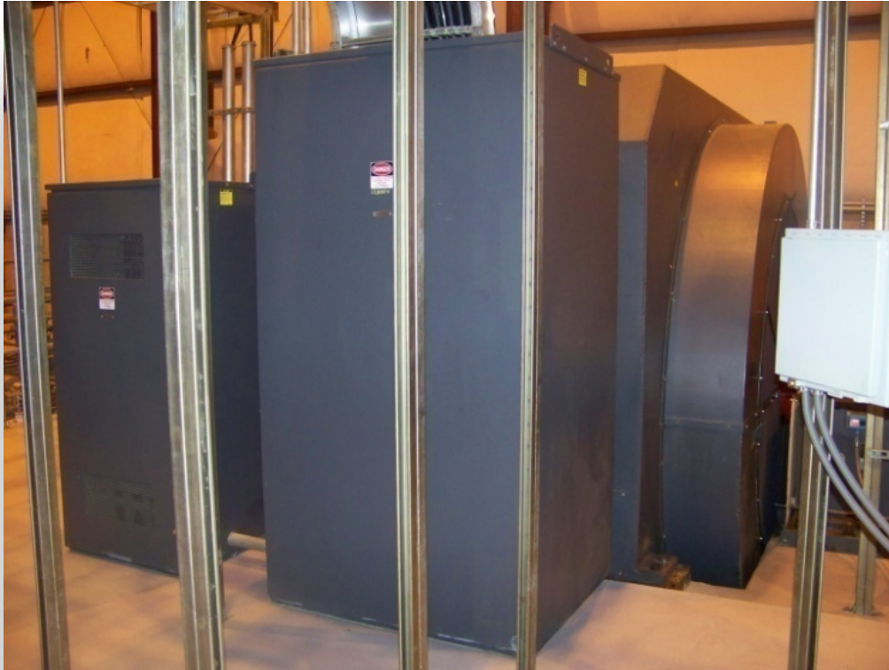
Generator Neutral High Resistance Ground Cabinet
