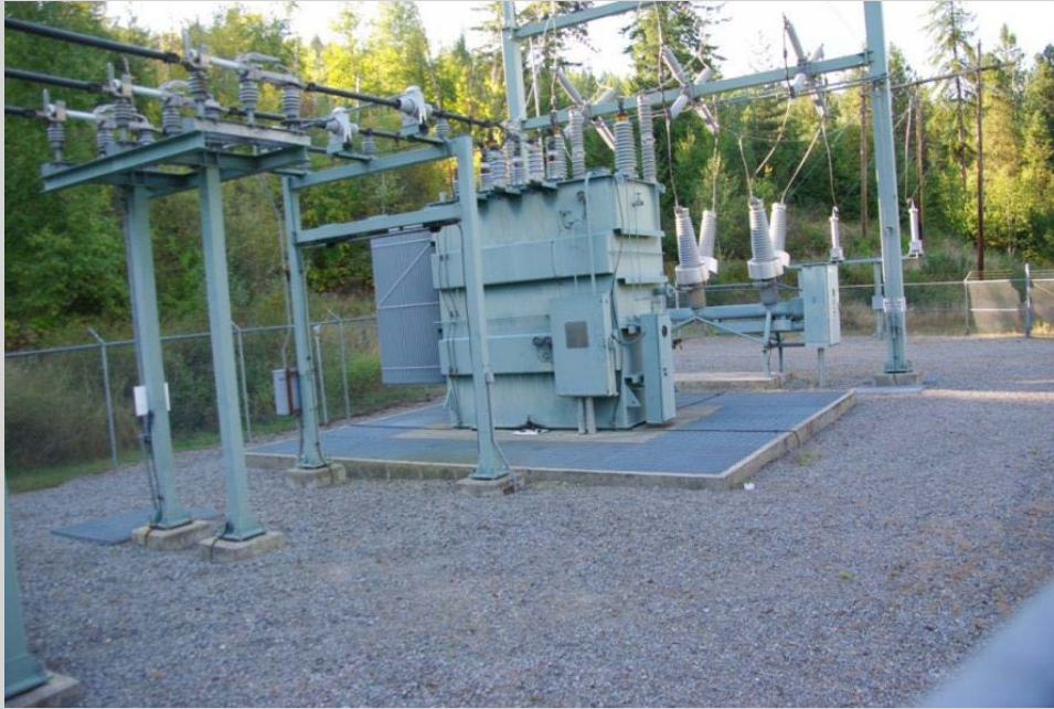
Substation and Generator Step-up Transformer
