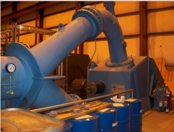
Unit 1 and 2 Typical Penstock Bifurcation for Upper and Lower Nozzle Flow Diversion
