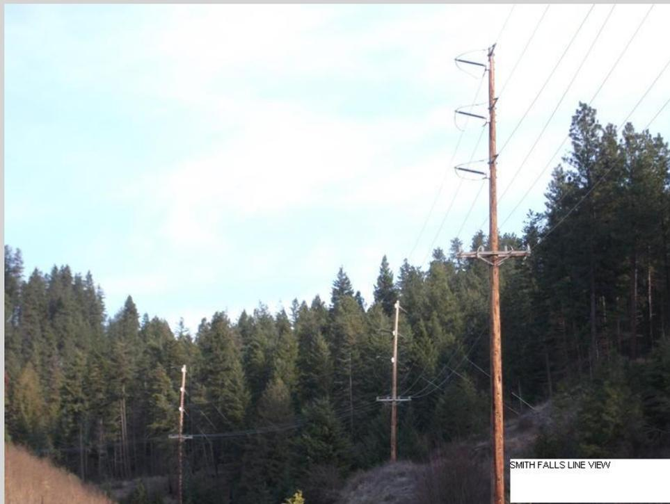
The most recent pole inspection was completed in 2010, with no notable findings and no internal decay detected. Testing included visual inspection of poles and attached hardware, sampling to determine effects from insect damage or decay, and treatment where required. There is a current project to relocate a tower at the crossing of the Kootenai River adjacent to the plant, which has shown signs of guy wire anchor erosion.
