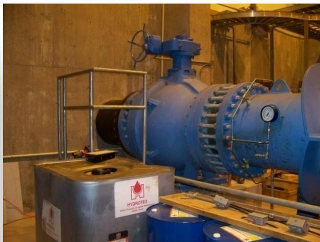
Typical Unit Penstock Penetration into Powerhouse
