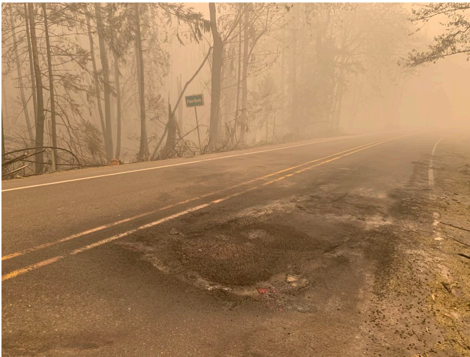
Road damage on Highway OR 126 during the Holiday Farm Fire in September 2020. Courtesy of Oregon Department of Transportation.
