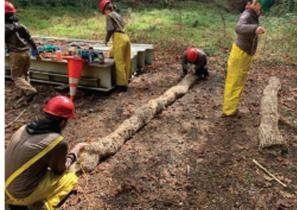
Photo 1. Straw wattles placed on a slope
