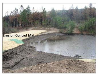
Photo 1. Erosion blanket example
