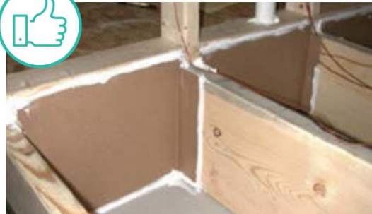
FLOOR JOISTS UNDER KNEEWALL (BLOCKED WITH RIGID MATERIAL AND SEALED WITH CAULK).
