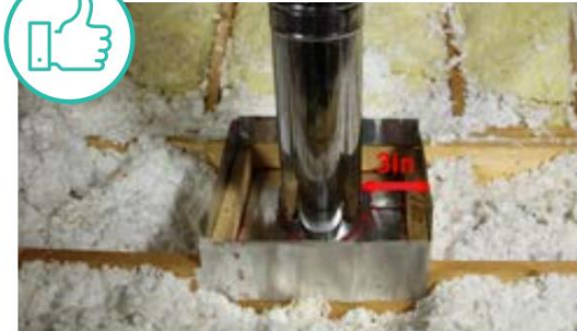
SEALED PENETRATION (HEAT-PRODUCING).
