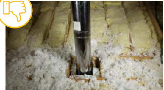
UNSEALED PENETRATION (HEAT-PRODUCING).
