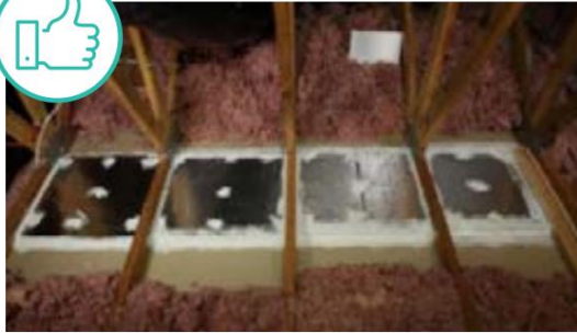
SEALED CHASE OR CAVITY.
