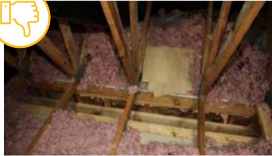
OPEN/UNSEALED CHASE OR CAVITY.
