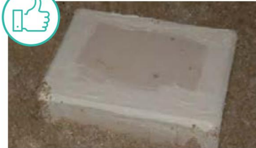
NON-IC FIXTURE WITH DRYWALL SHIELD (HAT).
