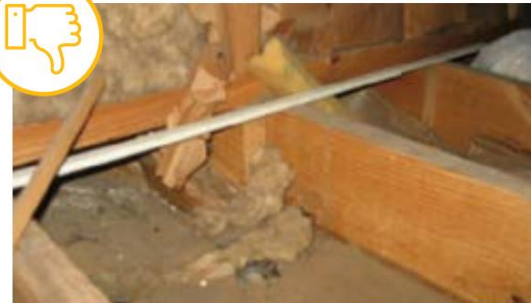
FLOOR JOISTS UNDER KNEEWALL (NOT BLOCKED WITH RIGID MATERIAL AND UNSEALED).
