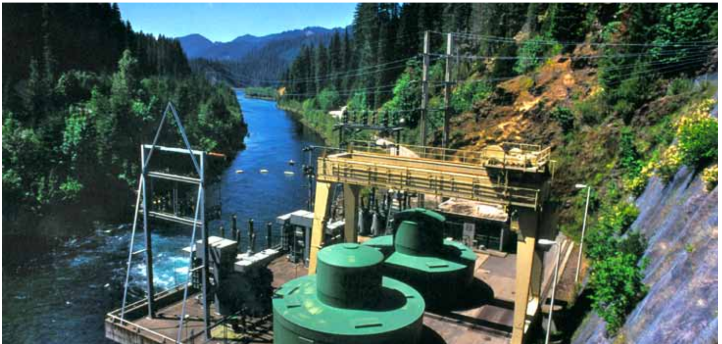
Carmen-Smith Power Plant
