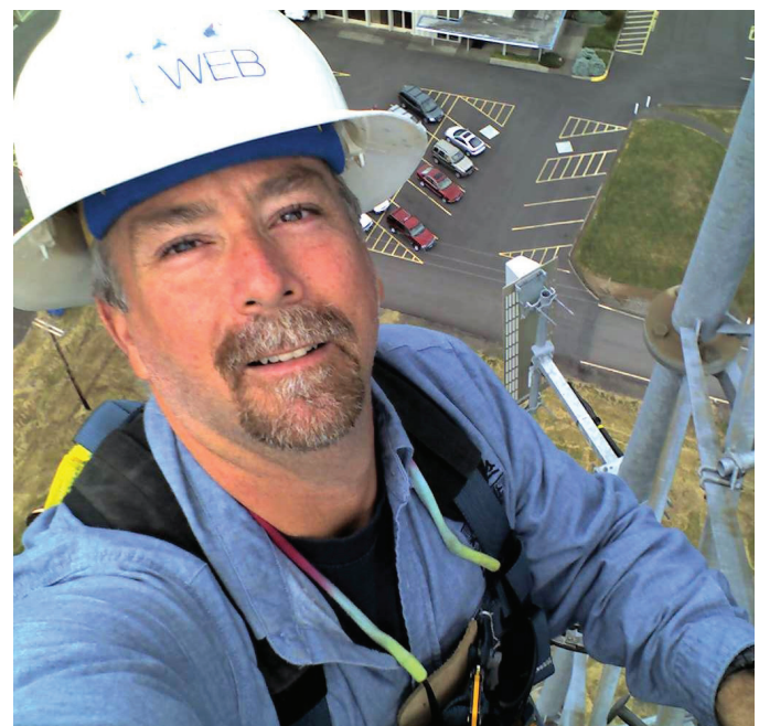
Electric line work
