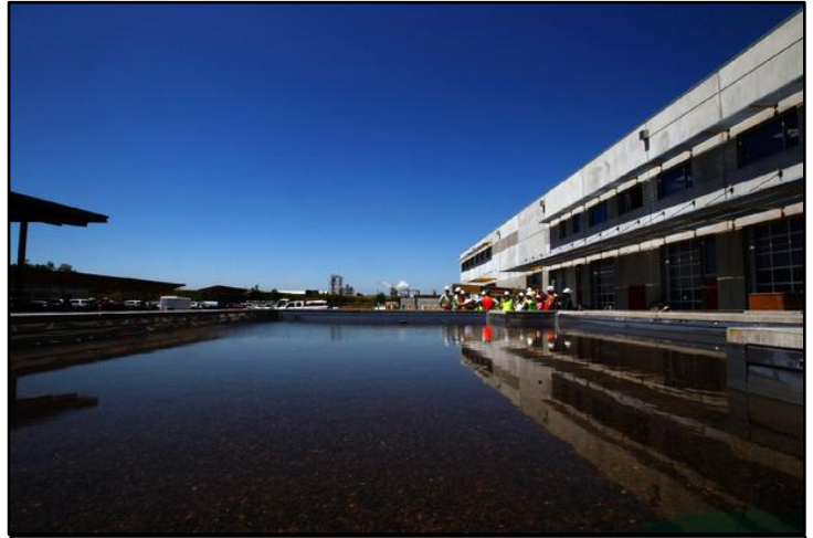
Kevin Clark/The Register-Guard. Water is reflected on the eco-machine at the Eugene Water & Electric Board's new Roosevelt Operations Center. The machine treats water and sewage on site.
