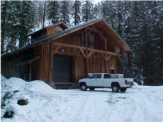
Figure 2: Picture of the Powerhouse
