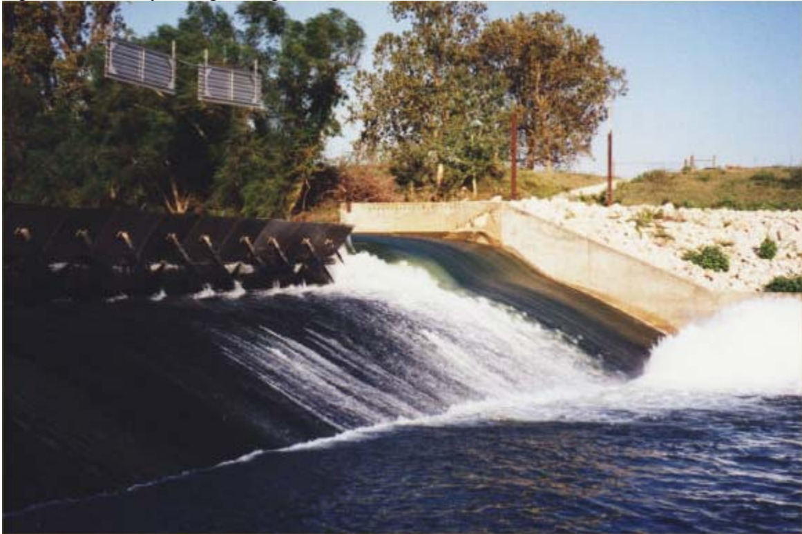
Figure 3 Obermeyer Regulating Weir – Downstream View
