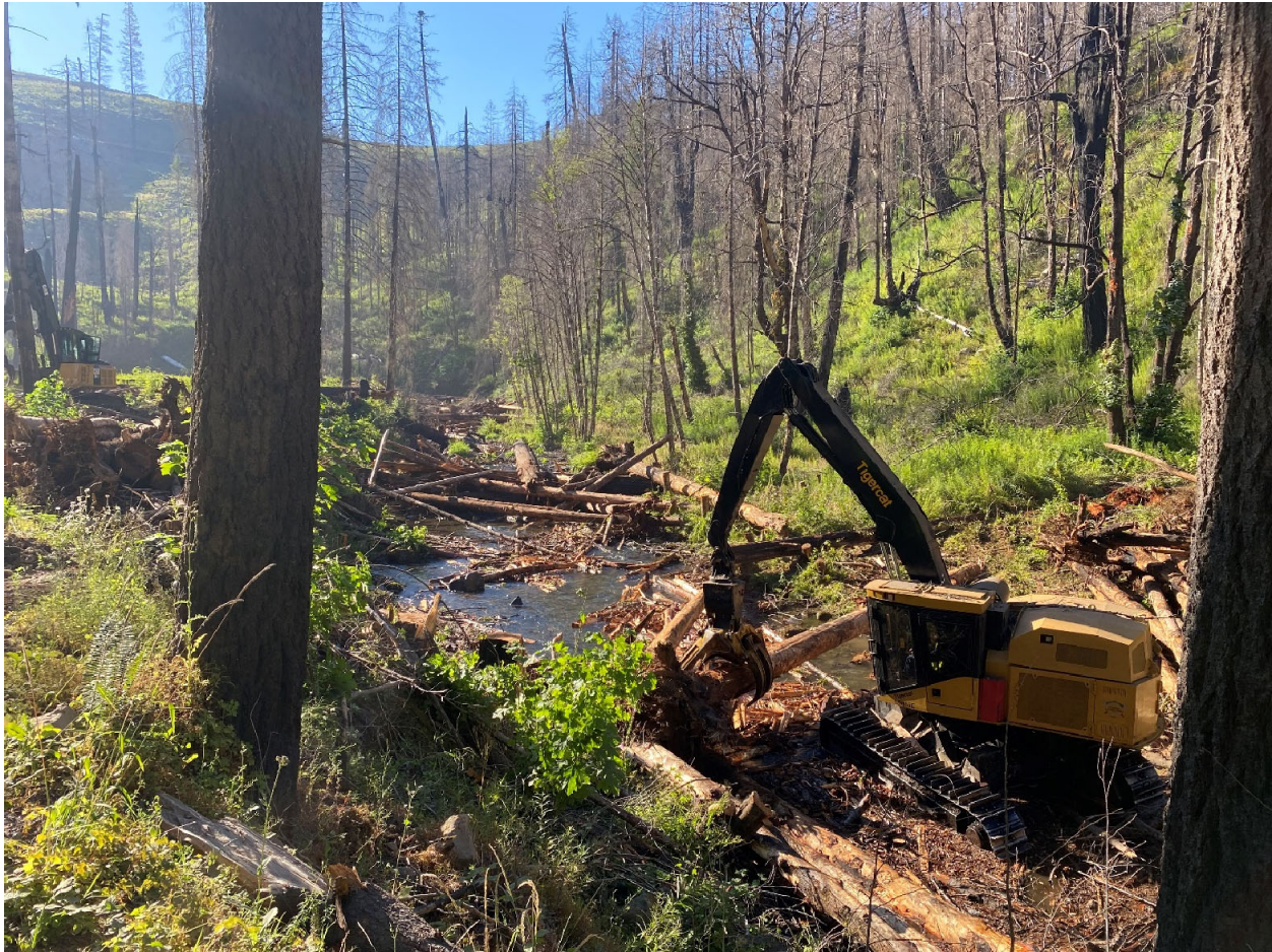
Figure 1-2: Gate Creek Large Wood Placement
