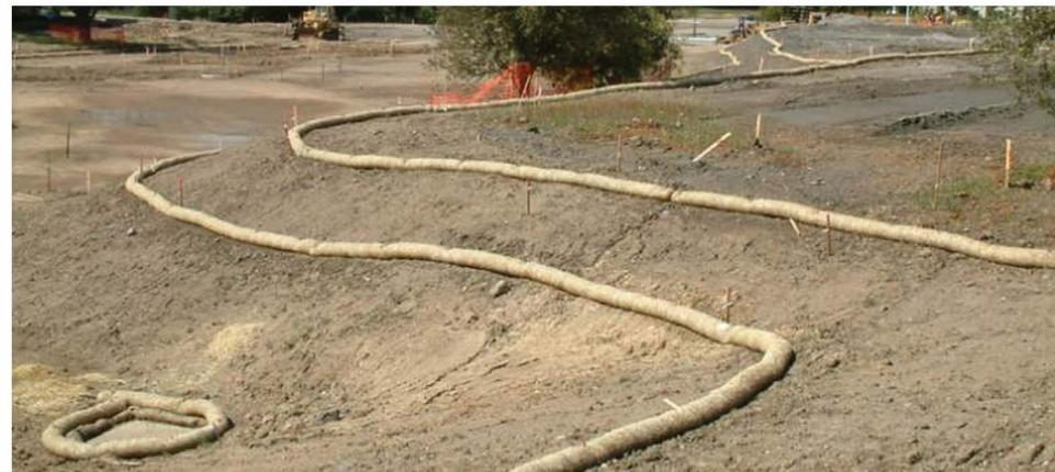
Photo 1. Straw wattles placed on a slope
