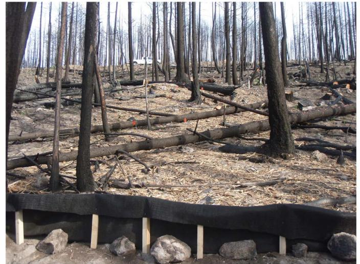
*Photo 1. Sediment fence installation*
