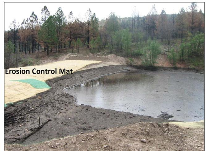
Photo 1. Erosion blanket example
