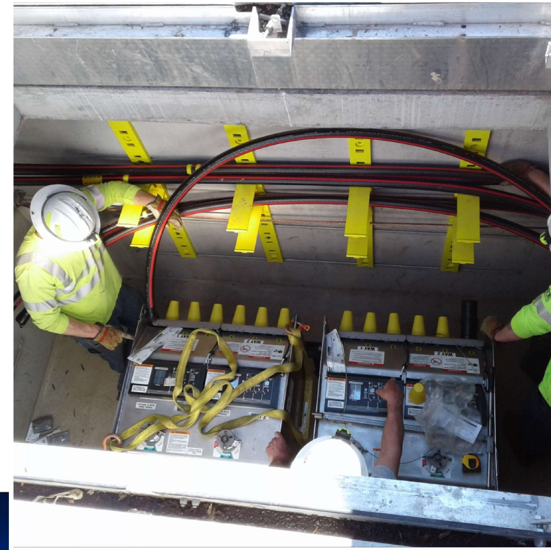
Eugene Downtown Underground Electrical Network Tie-Switch Installation
