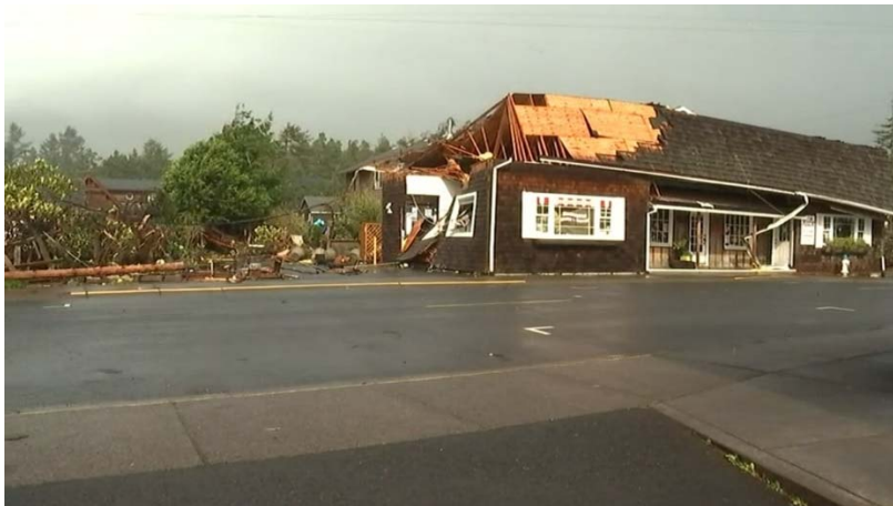
Picture 2-1. Source: KPTV-Manzanita, Oregon tornado damage October 2016
