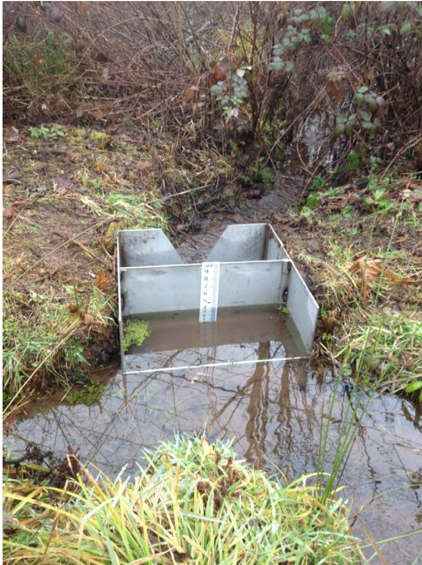
Figure 3. Permanent seepage weir monitoring station
