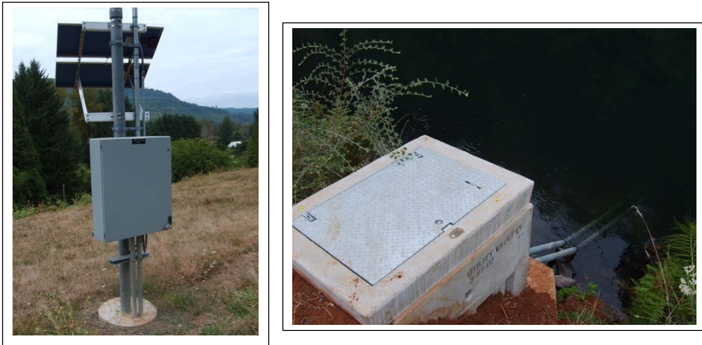
Figure 4. HMCS water level monitoring station, Leaburg Canal
